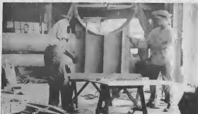
Boiler shop (5). Two boilermakers study the problem of repairing a saddle for an exchanger from one of the process units. Note plate roll in background which is used to curve boiler and tank plate.
